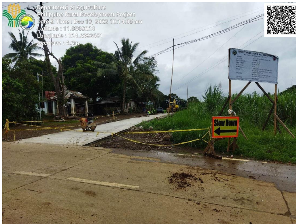
IMG 2 - Brgy. Donghol to Brgy. Mahayag, Ormoc City, Ongoing
