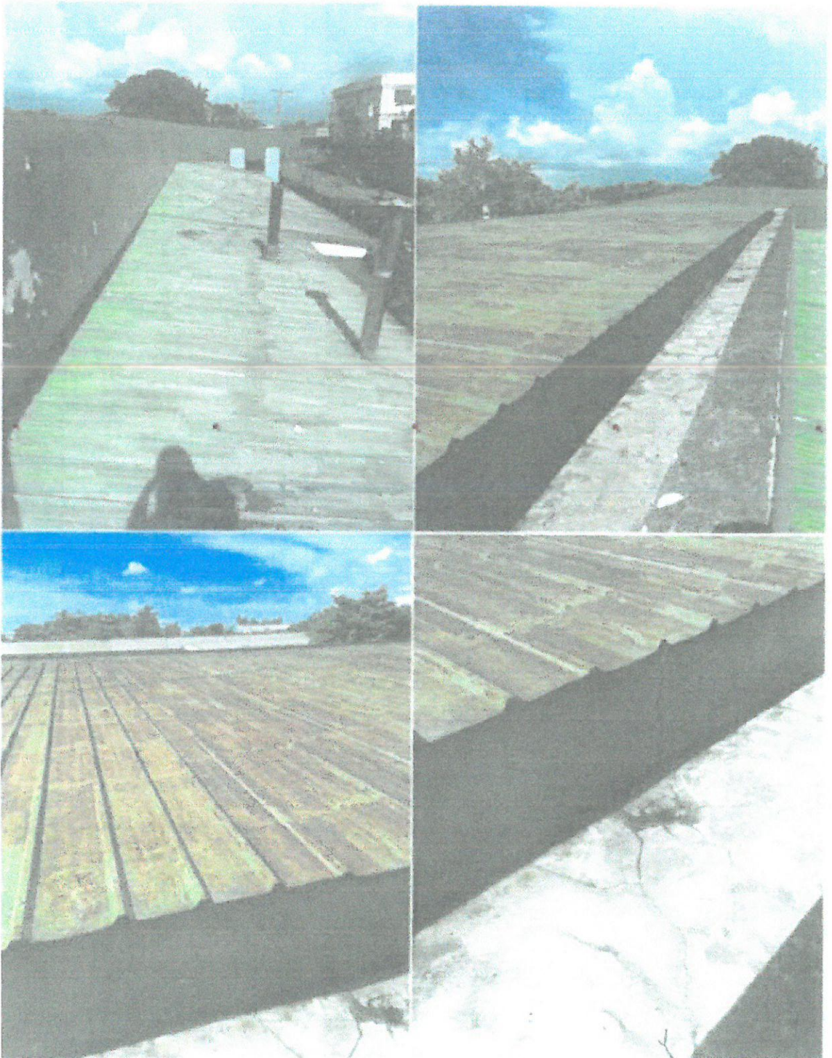
SOUTH BUILDING ACTUAL ROOFING
